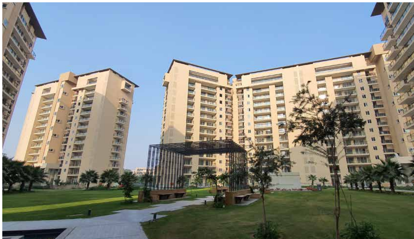
actual photograph of the JOI Phase - 01
